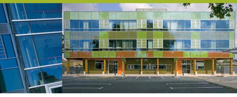
The composite curtain wall from AM Profiles features laminated pine mullions and transoms with aluminium cappings. The system offers cutting edge design, excellent value and breathtaking aesthetics. Large span and significant weight capabilities open up wonderful imaginative design possibilities.
